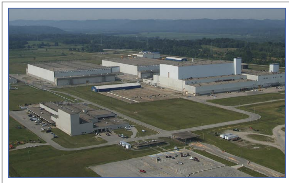
The American Centrifuge facility in Piketon, Ohio has an area of more than 25 football fields under roof
